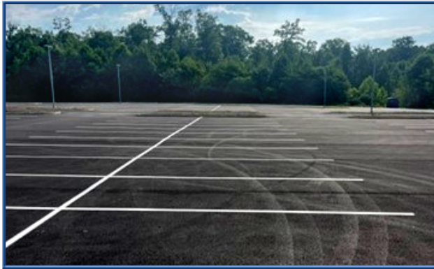
Catharpin Park Parking Lot Paving
