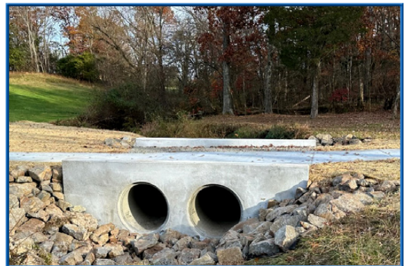
Prince William Golf Course Culvert Repair
