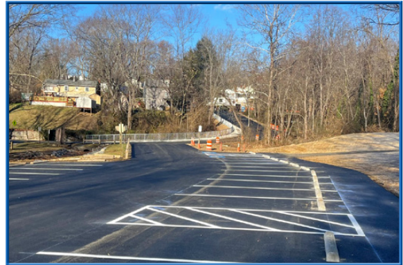
Cloverdale Park Site Improvements
