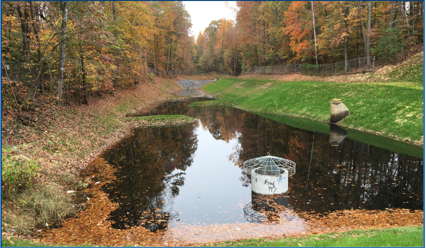
Powells Creek Watershed Water Quality Retrofit
