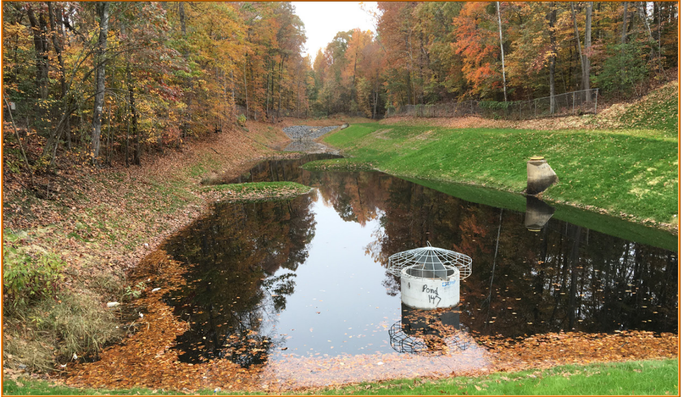
Powells Creek Watershed Water Quality Retrofit
